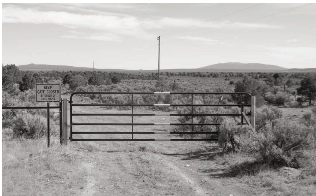
Fig. 1. A typical gate found along rural highways in New Mexico with open 10.16 cm diameter pipes functioning as anchors on both sides.
