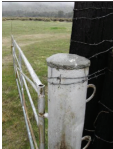
A cement cap is a simple and cost effective solution.
